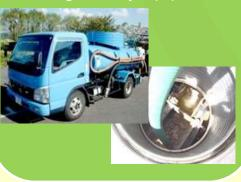
Visual Inspection Measure water level in the tank, scum, accumulated sludge, aeration mixing condition, returned water
